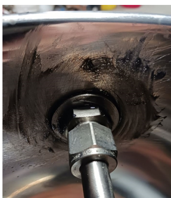
Internal Fitting showing seal of Belzona 2311
