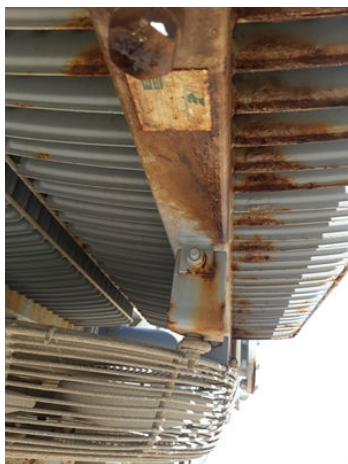
Initial condition illustrating rust and leakage.
