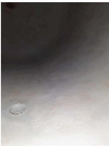
After surface preparation by grit blasting
