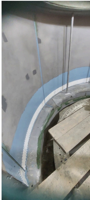
Rebuilding the pitted areas using Belzona 1311 and then applying Belzona 1391T as an adhesive to bond Belzona 9811 Almina Tiles
