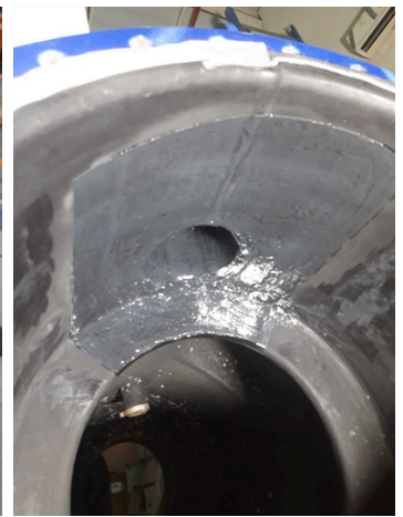
RUBBER LINING REPAIR COMPLETED
