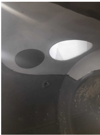
After surface preparation AND DURING SALT CONTAMINATION TEST
