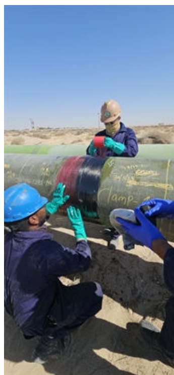
Application of Belzona Superwrap II
