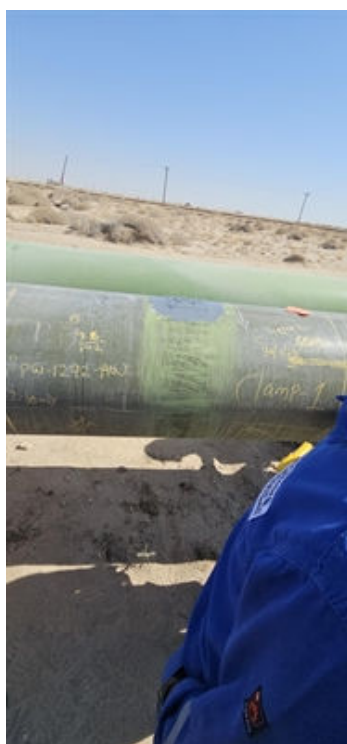
Steel plate bonded using Belzona 1212
