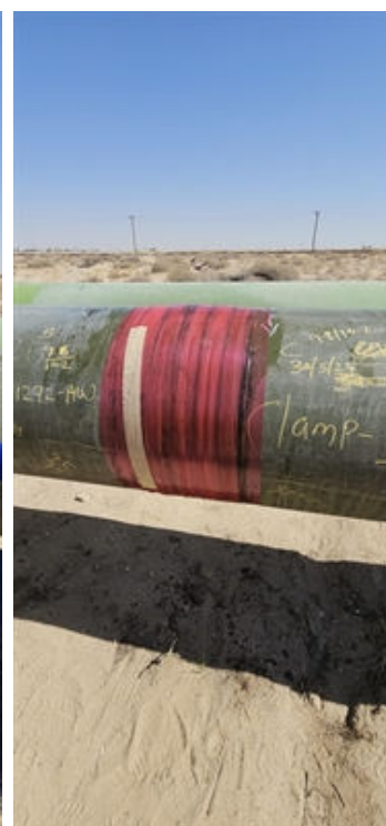
Completed Belzona Superwrap II repair
