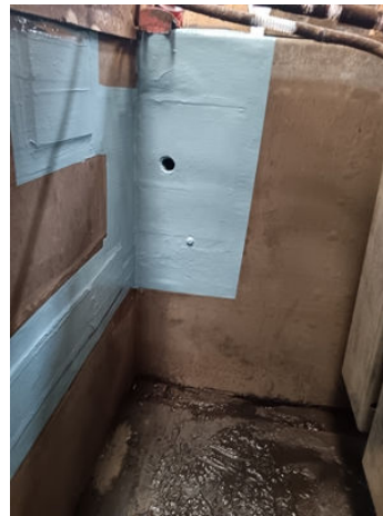
Second Coat Belzona 1391T
