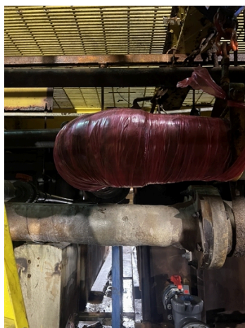
Newly installed Belzona Superwrap II
