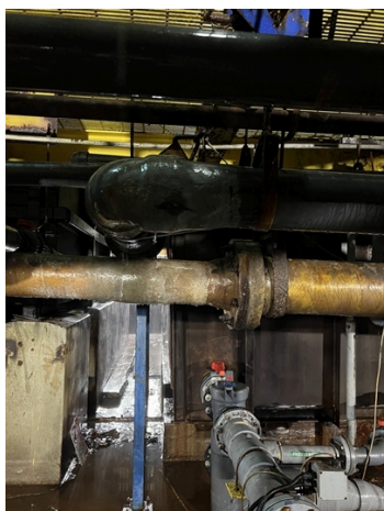
Failed fiber glass
