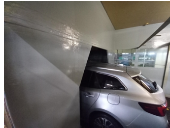
5 years on and the coating is still perfect. The client uses this as an example of their maintenance regime
