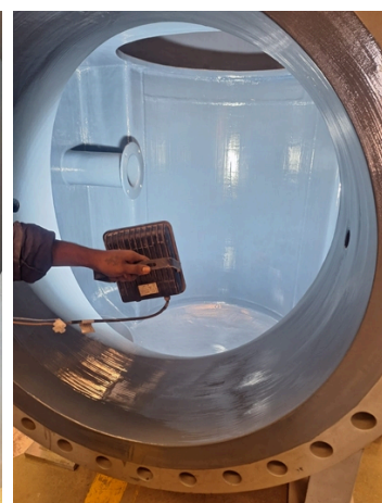
Completed application of Belzona 1311 & Belzona 1321
