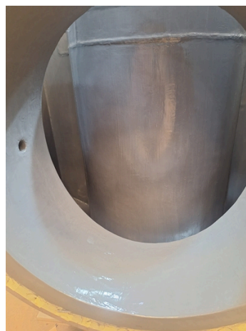
Belzona 1311 & Belzona 1321 application for the internal shell.
