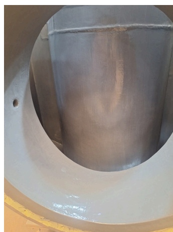
Belzona 1311 & Belzona 1321 application for the internal shell.
