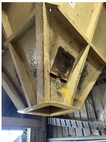
Tapered bottom end making bottom access difficult.
