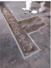
Damaged area prepared and conditioned with Belzona 4911 screeded and feather edged ready to accept Belzona 4131 MagmaScreed
