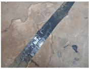
One of 5 expansion joints raked out, cleaned, conditioned with Belzona 2911 Conditioner and finished with Belzona 2211
