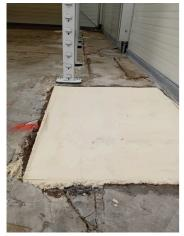
Uneven floor area made good using Belzona 4111 MagmaQuartz to support main racking stanchions
