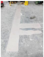
Damaged area fully repaired, with Belzona 4131 MagmaScreed to provide flat safe running surface for fork lift Hi-Build elastomer trucks and handling machinery
