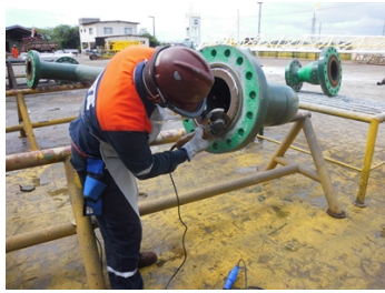
Surface preparation on the groove
