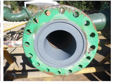
Flange face repair complete and ready to put back in service
