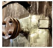
Manual preparation of the C.S. The cracked steel shell was tank shell removing all contaminates and creating a cross-hatch profile for adhesion.
