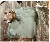
mixed and applied Belzona 1511 Hi-temp, filler to smooth over the prepared area in readiness for the application of onto the steel Tank Shell. Belzona 1983 SuperWrap II
