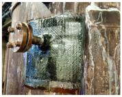
The completed SuperWrap II (1983) patch bonded in place over the Belzona 1511 and
