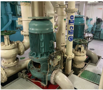
External photo of the Fire and Bilge Pump in Service
