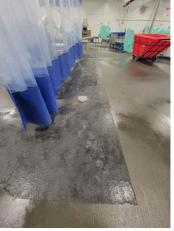
The floor was prepped with hand tools, cleaned and then repaired whit Belzona 4111.
