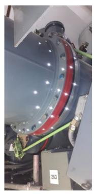
SF6 leaking from multiple location around pipe joint. Client covered joint with tape to stem leak.
