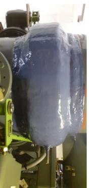
SF6-FIX leak sealing repair completed, with vent pipe left open at 6 o'clock position until 5x layers of Belzona 9371 using full cure is achieved. Vent pipe Belzona 1981 resin for wetting. is capped off following full cure.
