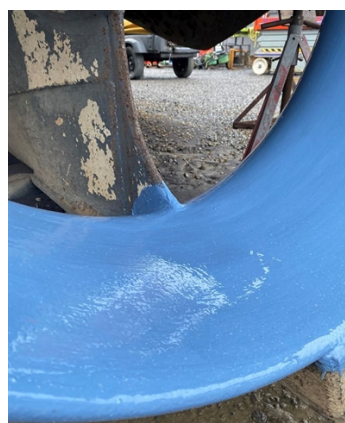
Close-up look at the coated areas once the job was completed
