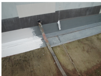
Belzona 3921 applied & 1st coat of Belzona 3131
