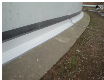
1st coat of Belzona 3131
