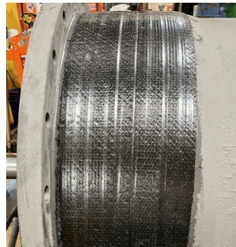
Exterior of diffuser reinforced with Belzona Superwrap II System
