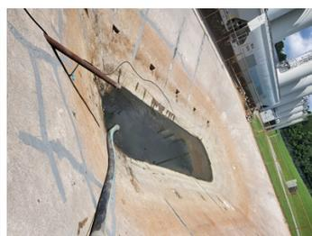
Cracks being repaired with Belzona 3121
