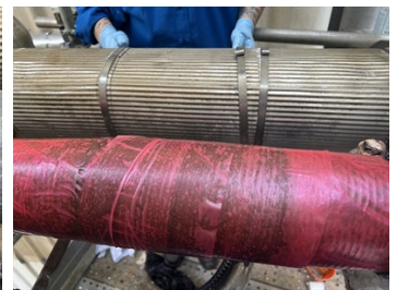
After application of SuperWrap II system.
