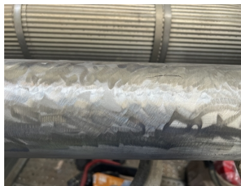
Pipe after surface preparation
