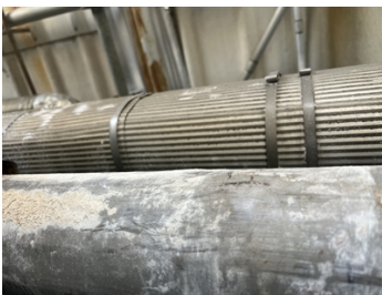
Pipe before surface preparation.
