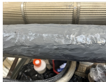
After application of Belzona 1212.
