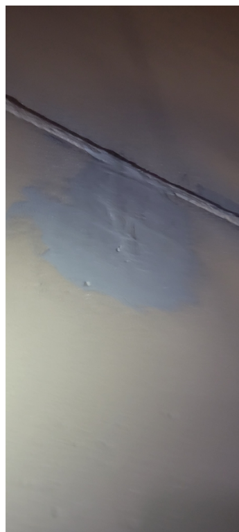
Belzona 1121 applied to fill in the pits.
