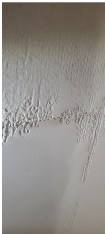
Pitting caused by corrosion at the inside of the water storage tank.
