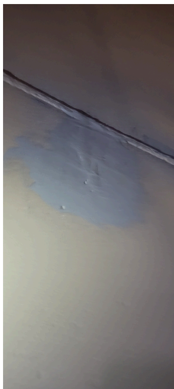
Belzona 1121 applied to fill the pits.
