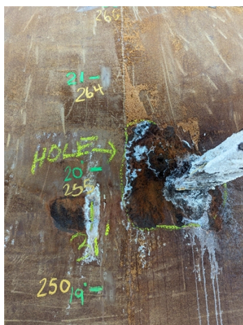
Close-up of corrosion.
