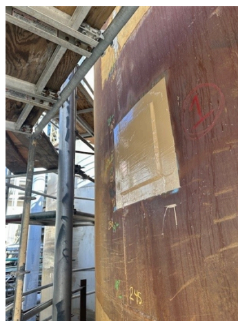
Close-up of finished application of plate bonding.
