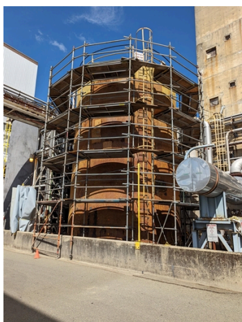
Tank experiencing corrosion.
