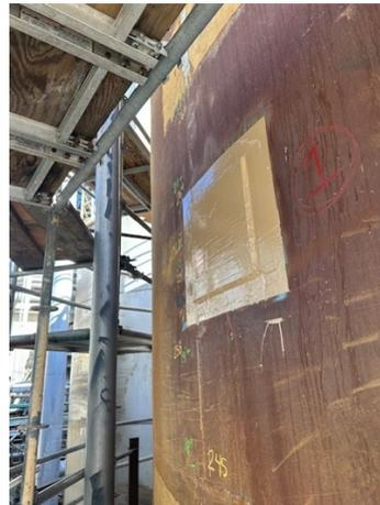
Close-up of finished application of plate bonding.
