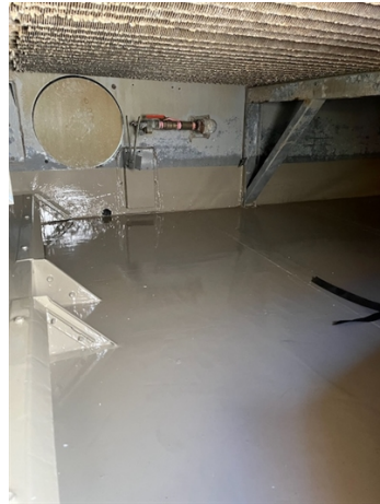
First coat of Belzona 5815 beige.
