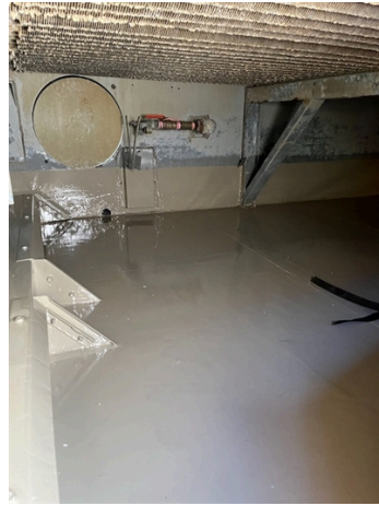
First coat of Belzona 5815 beige.
