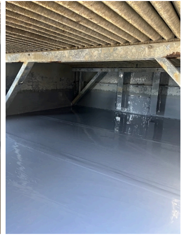
Second coat of Belzona 5815 grey.
