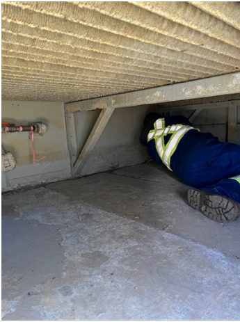
Previous coating system.
