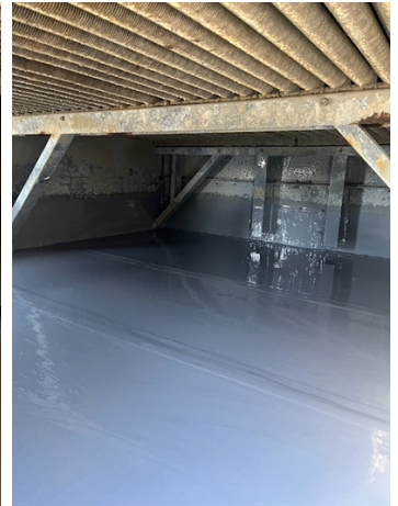
Second coat of Belzona 5815 grey.
