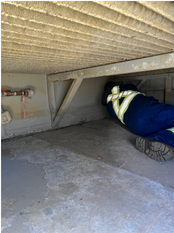
Previous coating system.
