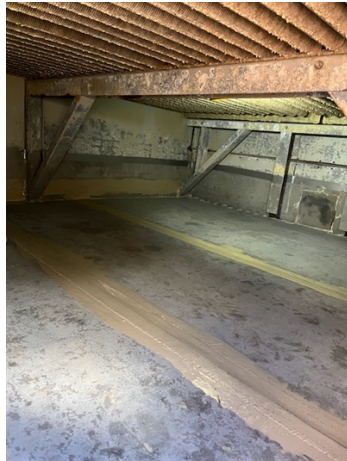
Belzona 9371 fibreglass strips wetted out with Belzona 5815 to bridge joints.
