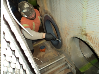
Picture showing the application of the Belzona 1321.
