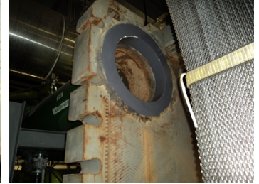
Picture showing completed application both coats of Belzona 1321.
