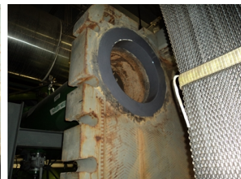
Picture showing completed application both coats of Belzona 1321.
