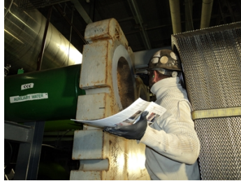
Pictures showing the application of Belzona 1111.
