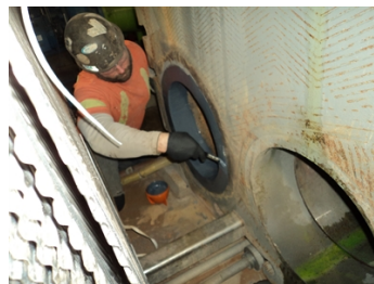
Picture showing the application of the Belzona 1321.
