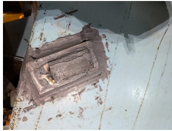
Belzona 1212 used to bond plate.
