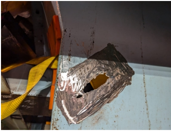
Hole prepared for repair.
