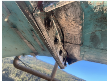
Surface preparation completed
