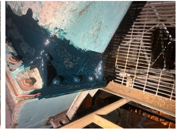
Coated with Belzona 2141 for longevity
