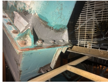
Rebuilt with Belzona 1311
