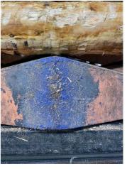
Steel grit blasted at welds that Belzona 1818 ready to be used. Belzona 1818 applied. would frequently wear away.
