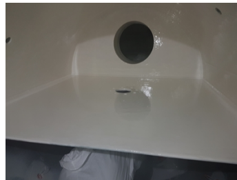
Full coat of Belzona 1331 being applied
