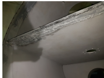
Repaired divider bar
