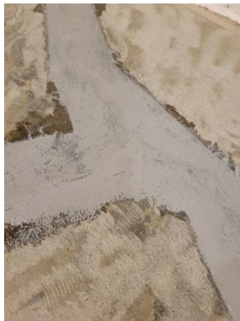
Crack was conditioned with Belzona 4911 and repaired using Belzona 4111.
