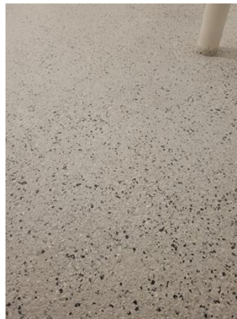
Vinyl flakes applied onto Belzona 5231.
