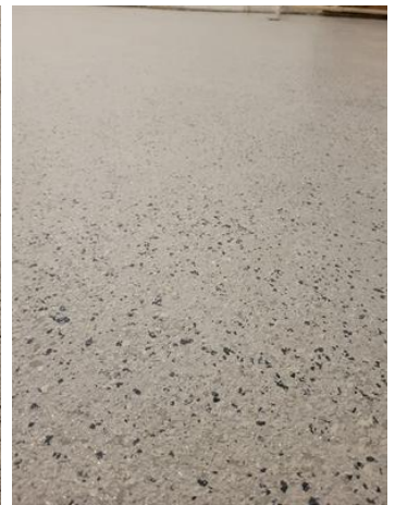
Belzona 5233 was applied as the clearcoat topcoat.
