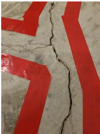
Repair area was defined.
