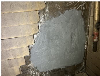
Holes repaired and ready for tile
