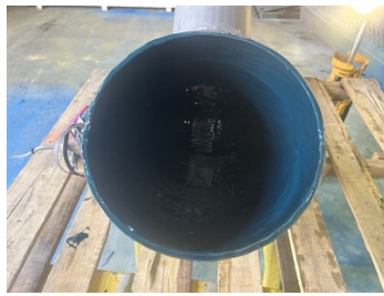
Base coat applied
