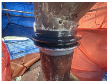
Belzona elastomer and cloth applied
