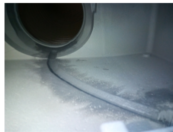
The missing original material was supplemented with the Belzona 1511 product.
