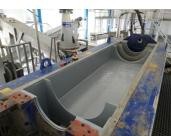
Corrosive damage to the gutter. Before applying Belzona
