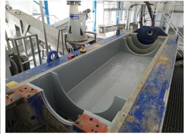
Corrosive damage to the gutter. Before applying Belzona products, it was necessary to blast the gutter.
