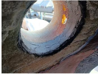
Filling the original missing material with Belzona 1111
