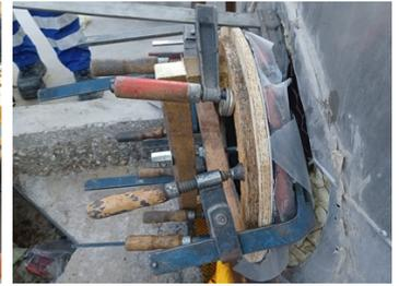
An auxiliary structure had to be built to repair the flanges.
