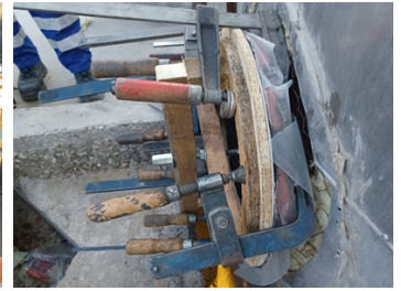
An auxiliary structure had to be built to repair the flanges.
