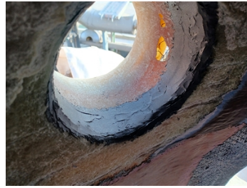
Filling the original missing material with Belzona 1111
