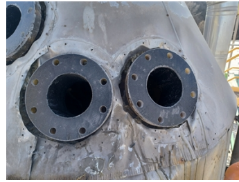
Repaired flanges and necks - ready for use
