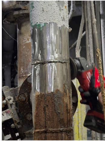
Removing the rust and pulp fiber and roughening the surface.
