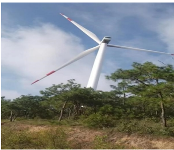
Full view of wind turbine
