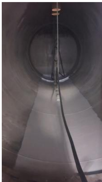
Blasted tank bottom.
