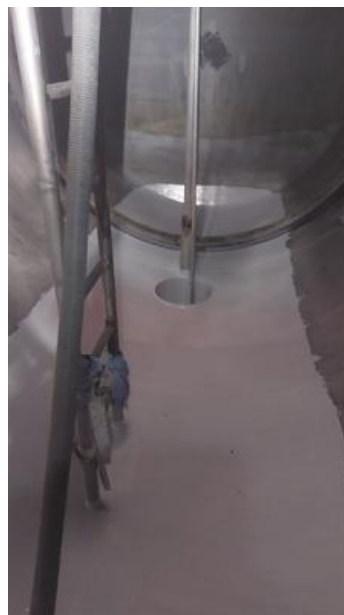
Application of the product Belzona 1391 T in two layers.
