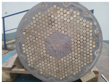
The repair was done using cork plugs.
