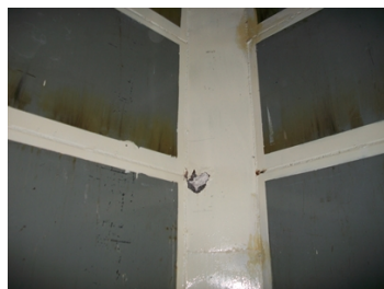
Corroded area
