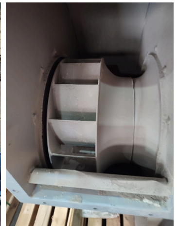
Fan wheel before repair
