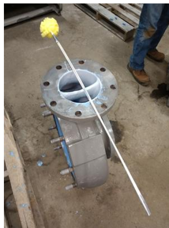
Applying the second coat of Belzona 1341.
