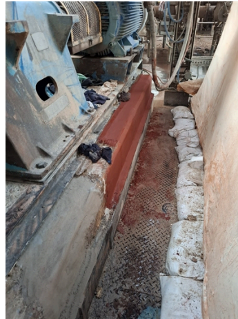
Application of Belzona 4181
