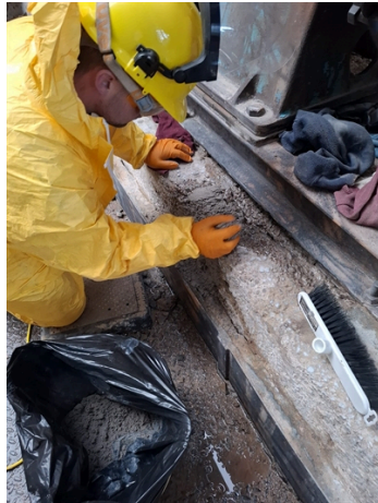
Application of Belzona 4131
