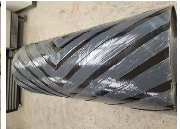
Belzona 2211 second coat
