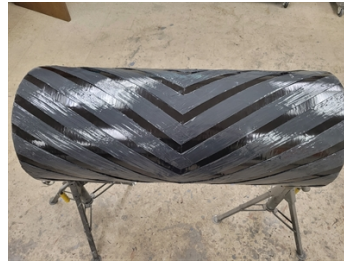
Belzona 2211 first coat
