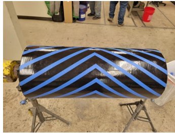
Demarcation on pully for Belzona application
