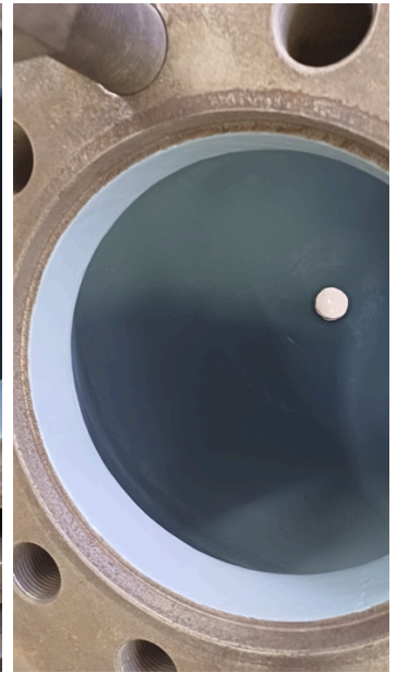
After coating with Belzona
