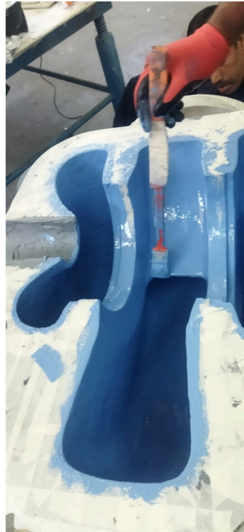
Coating application to the cutwater
