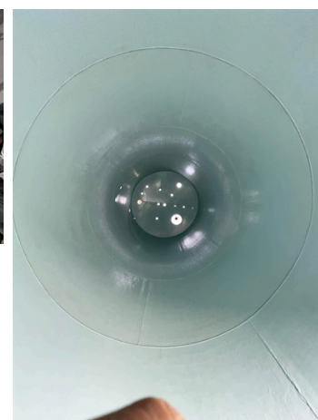
Final phase with Belzona 1593
