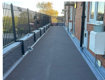
Balconies fully coated with the addition of Belzona Surefoot aggregate
